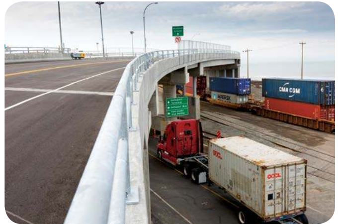
Completed overpass with a view of truck and train traffic
